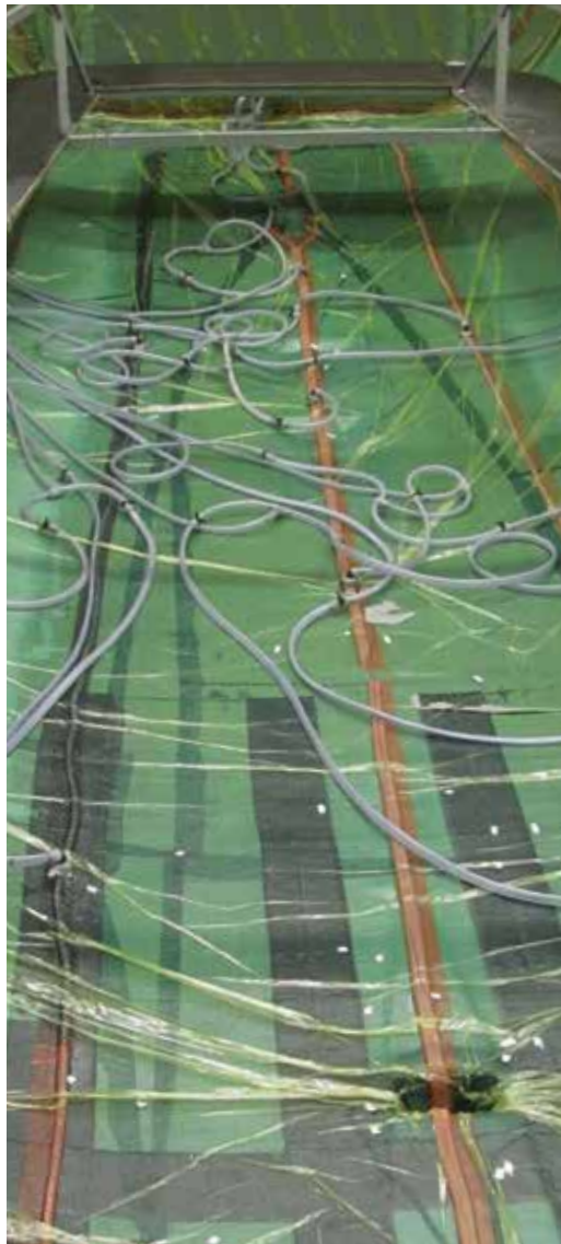
Vacuum infusion build of an Xperformance hull, showing uni-directional carbon tapes in hull laminate
